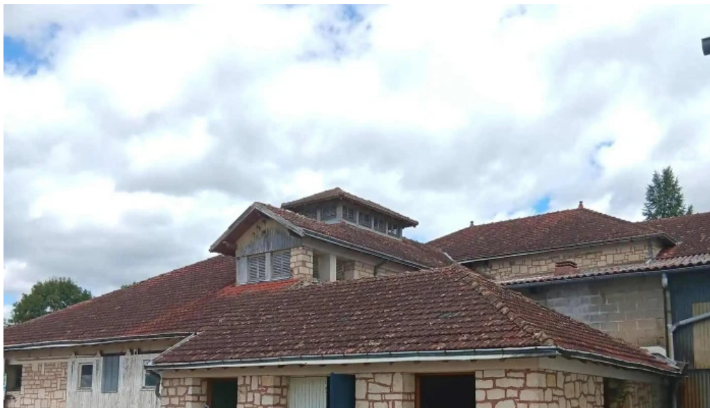
Laiterie cooperative darchigny archigny
